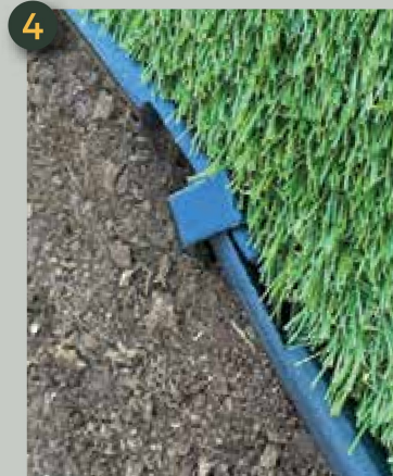
4 When the install is complete, all that should be seen in the head of the anchor stake
