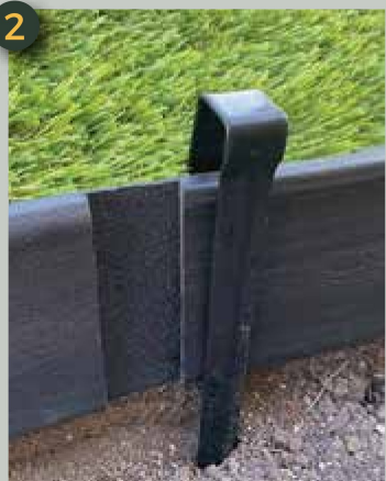
2 Leave 1 ¼" gap for expansion/contraction of the plastic
