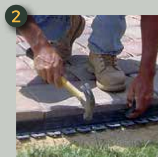
2 Slide the bottom section of the restraint until it is flush with the sidewall.
