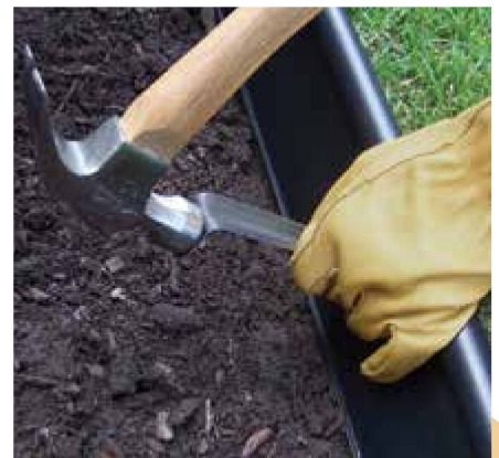
Secure into place with metal anchors
