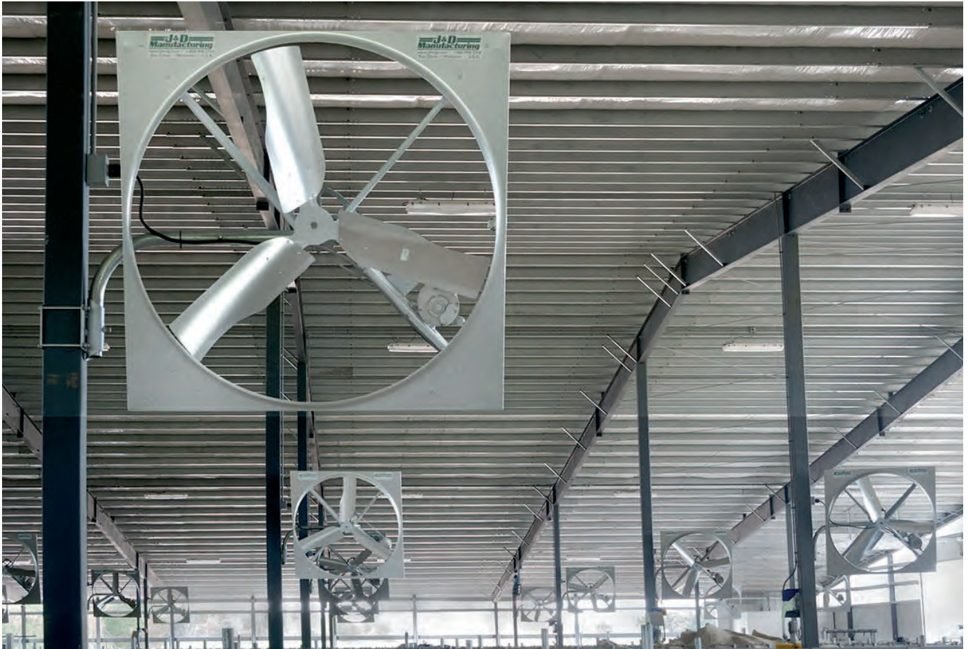
Belt Drive Panel Fans with Galvanized Prop and VRSBRSQ6X Swivel Offset 6" Square Column Mounting Brackets
