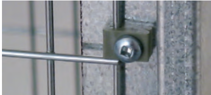
Poly guard clips to reduce vibration for quiet performance.
