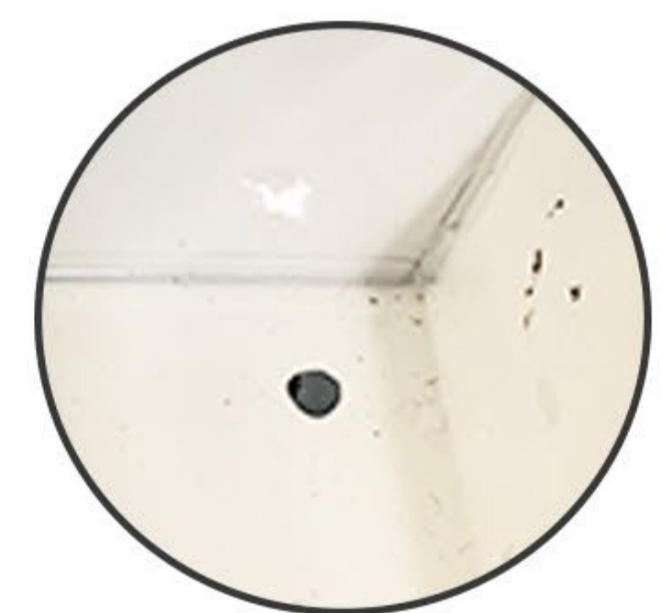
Four Drain Holes
