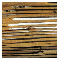
CARPENTER ANT DAMAGE
