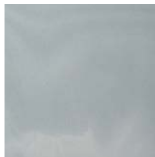
Weathered Concrete Ref: 92
